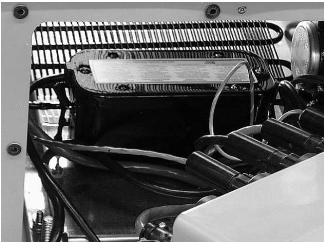
Figure 2: Positioning the Battery
